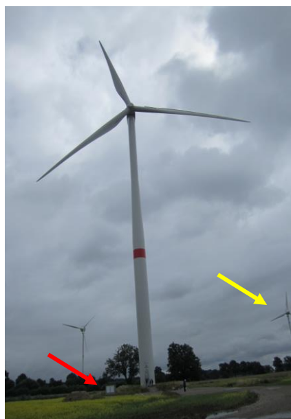
Figure 10: View of the transformer box at the foot of the wind turbine (red arrow left) and two wind turbines in the background (yellow arrow right: 404 m from the camera position).
